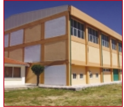
The new Gymnasium of the primary school in the village of Stimanga, Greece
